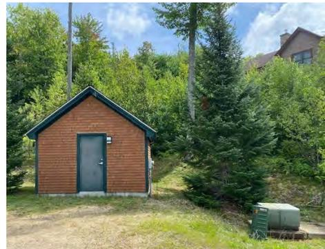
This pump station was built during the Cascade Ridge Subdivision development in 2005. The station contains two pumps used to boost water pressure to several properties located on Bean Bender Road.
